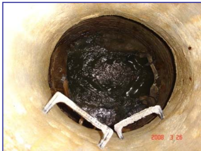
Manhole inspections provide insight into pipeline conditions in the project area.
